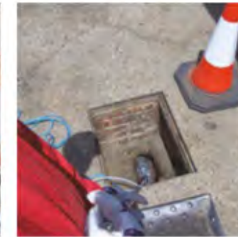
2. Pump up the bladder until fully inflated
